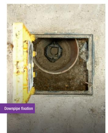
An incorrectly positioned surface box makes operation of the valve difficult or even impossible.
