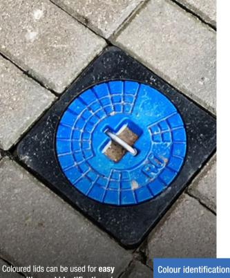
recognition and identification of an underground valve or hydrant. AVK offers surface boxes with coloured cast iron lid (epoxy coated) and coloured synthetic lid.
