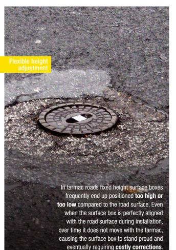
Due to the flexible top part of the AVK height adjustable surface boxes, a **perfect installation** is easy. The floating top part ensures a **safe and lasting alignment with the road surface** avoiding costly and time consuming corrections after installation.
